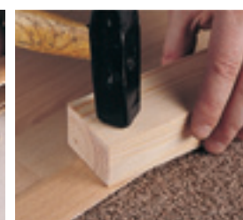
4. Hammer in with protecting batten
